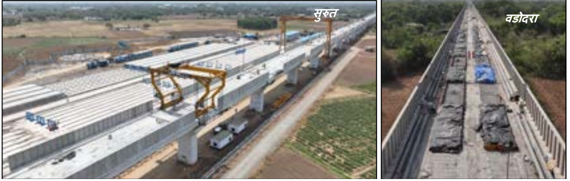
Noise Barrier Installation Work in Progress, Gujarat
